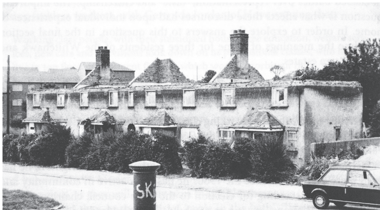
«Brighton. Whitehawk Road being demolished, 1980.» (Jones, 2012)
