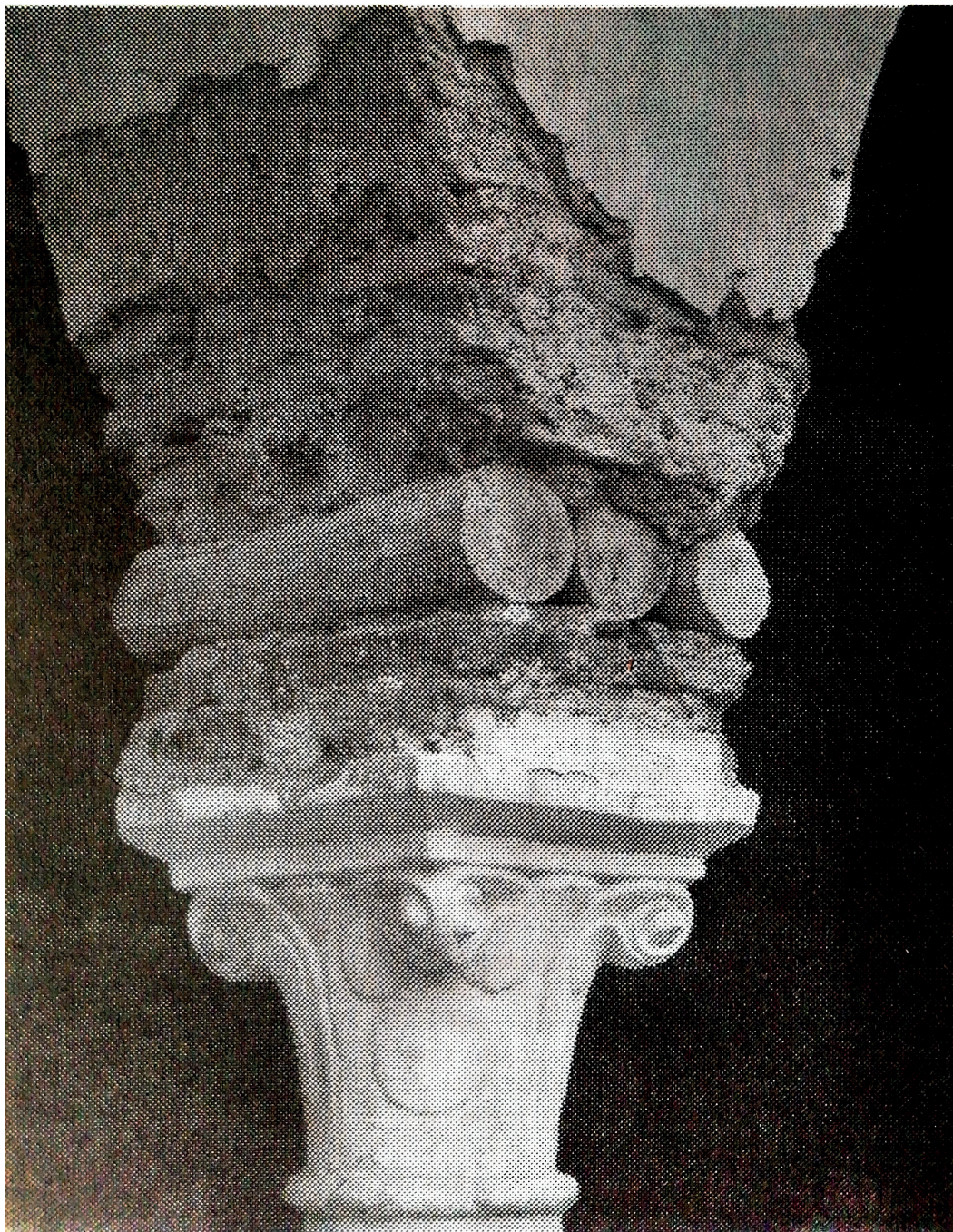
Layer of cedar on top of a column. Palace of the Dey, Citadel of Algiers (All rights reserved to Abdessemed-Foufa, 2005, Amina Abdessemed-Foufa, "Historic Earthquake-Resistant Constructive Techniques Reinforced by Wooden Logs in Algeria" (Lab ETAP, Institute of Architecture and Urban Planning, University "Saad Dahlab" of Blida 1, n.d.).)
