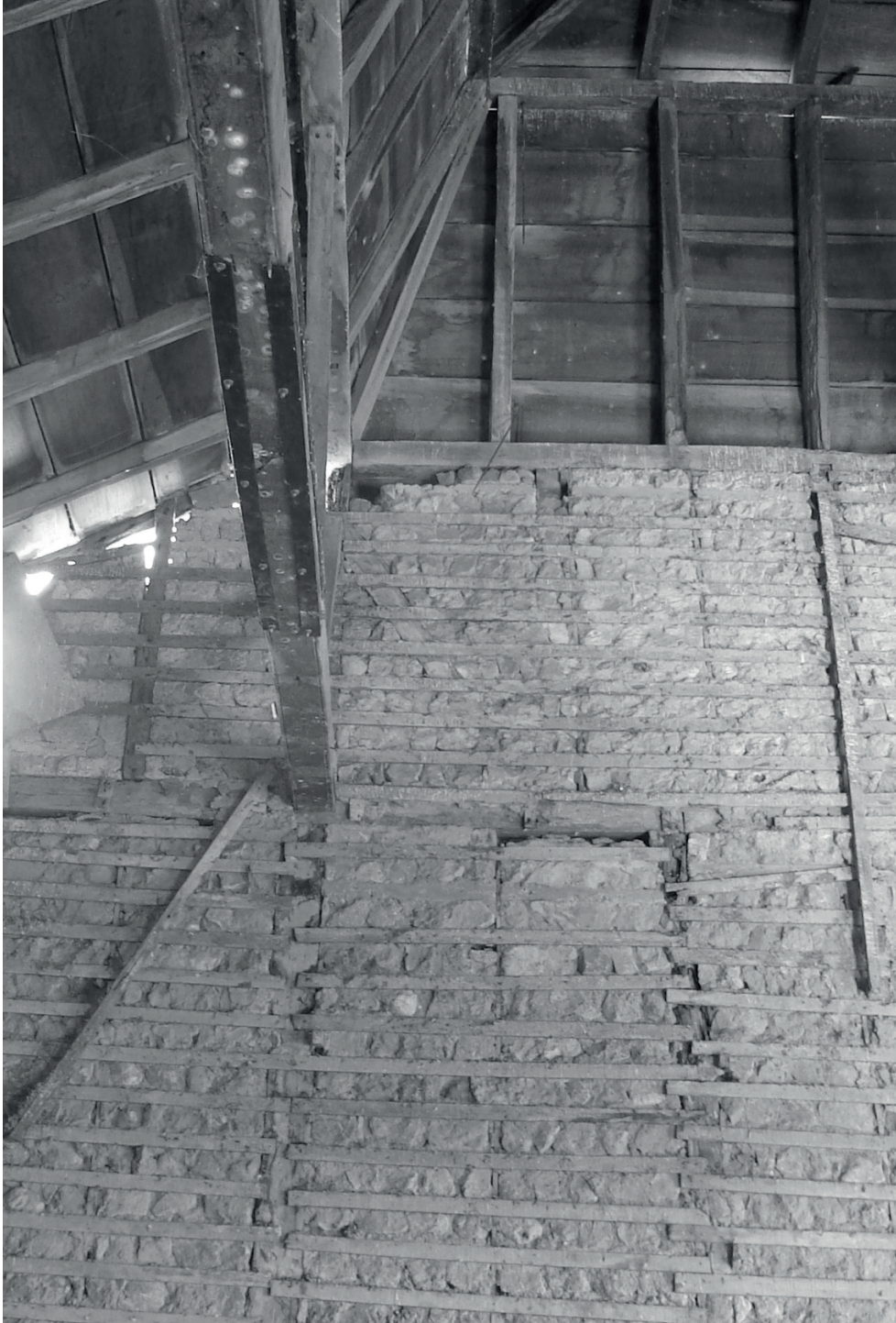
Wattle and daub wall (similar to Quincha, it's called "Taquezal" in Granada, Nicaragua (photo credits to Luis Fernando Guerrero Baca, 2008)
