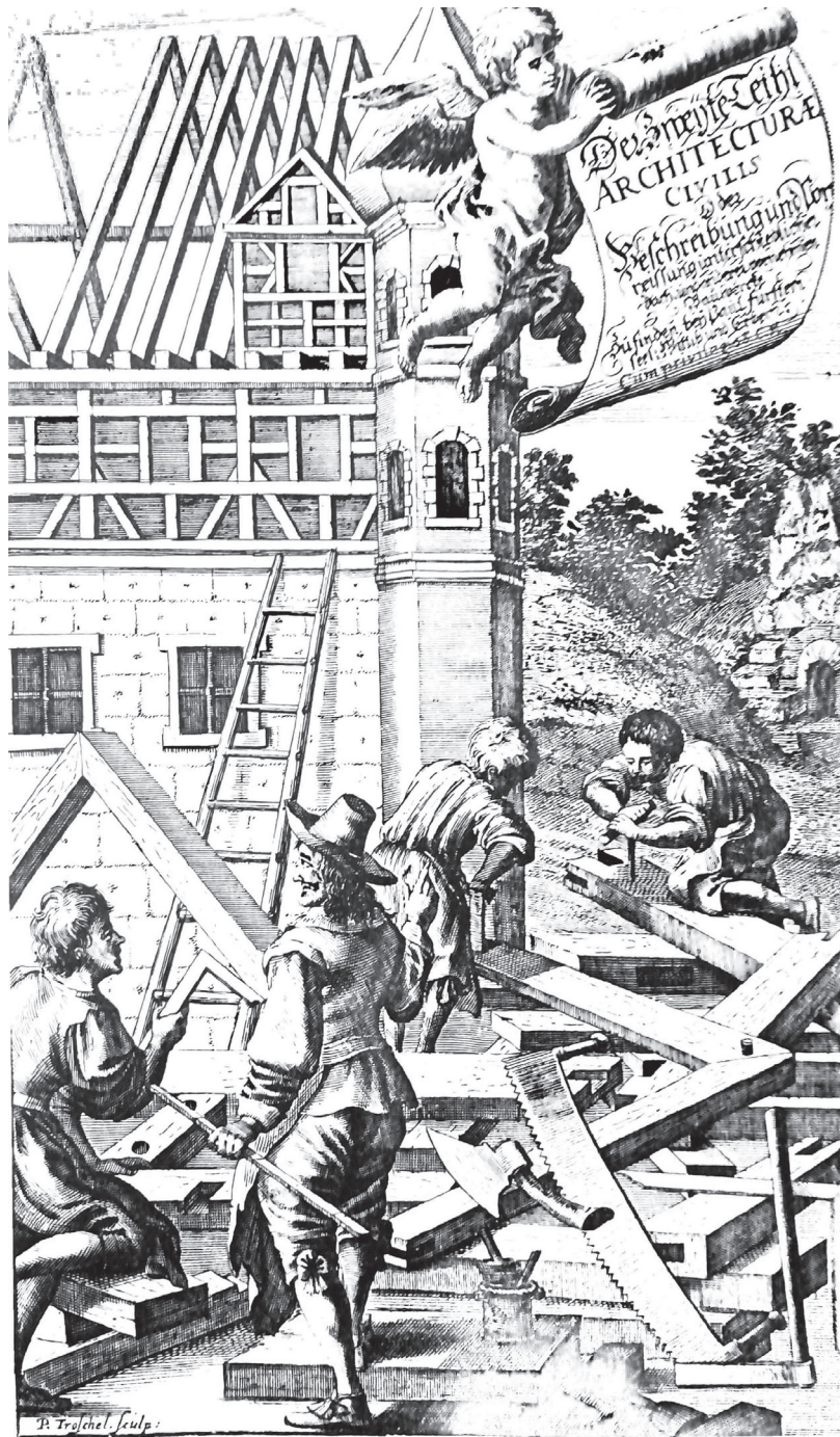
J. Wilhelm, building site of a Fachwerk house, 1668
