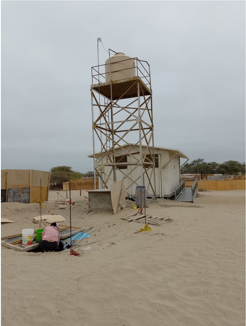
Water tank in original School in San Pablo village, 2022 | Lucia Gherzi
