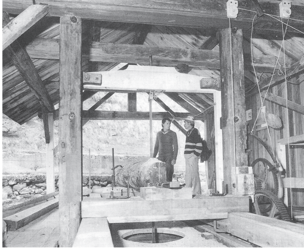
Fig. 50: Hydraulic saw and mill restored for the community in Sarreyer. © Jean-Marc Biner
