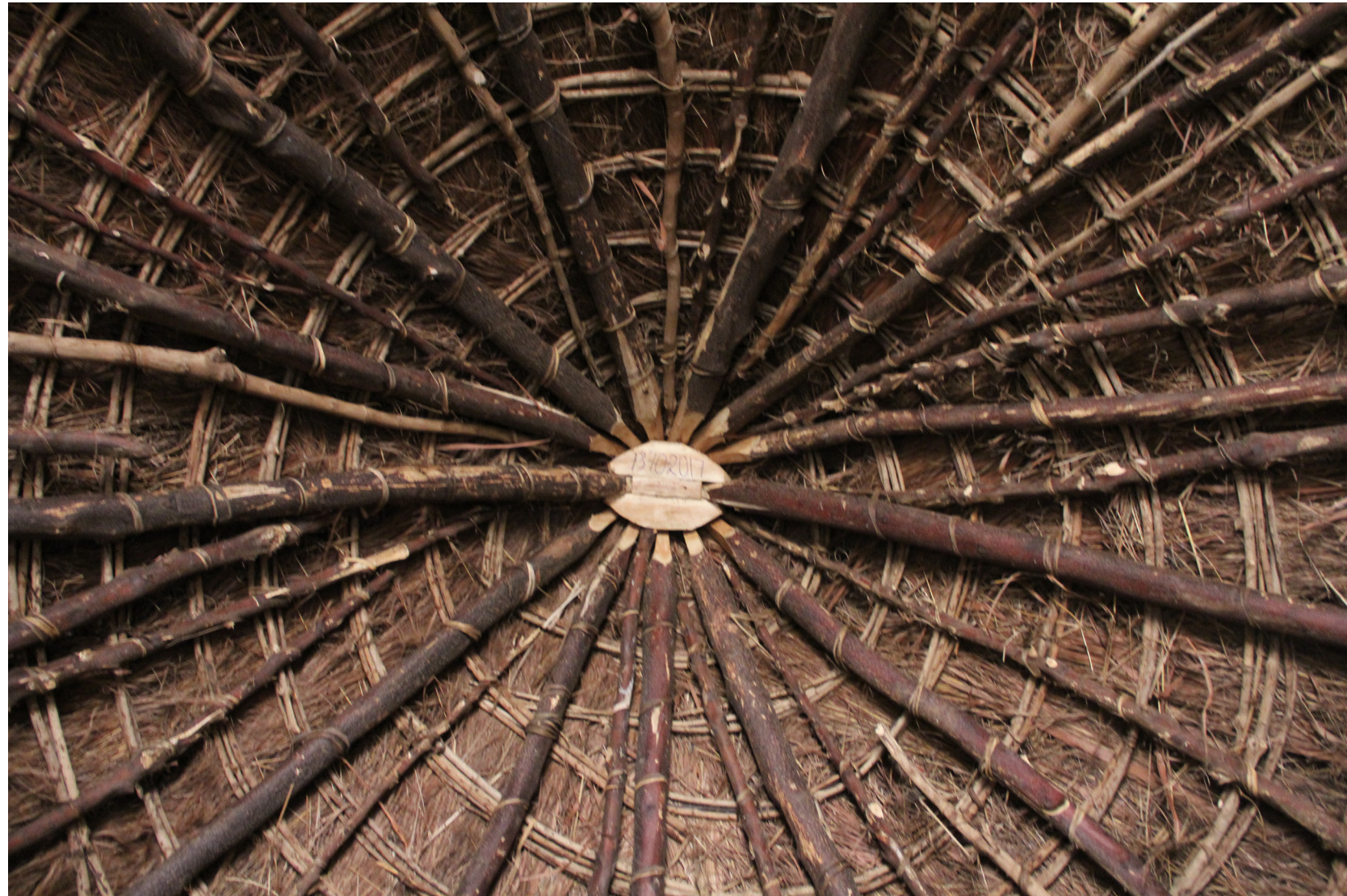
Detail: central connection of Roof structure This is the interlinking central element in a bigger hut (4m diameter).
