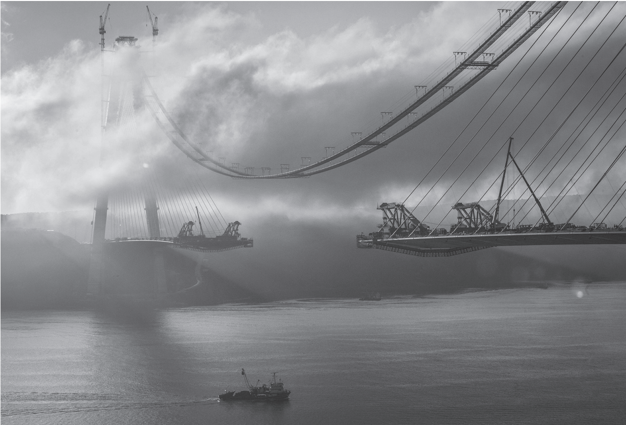
Construction of Yavuz Sultan Selim Bridge
