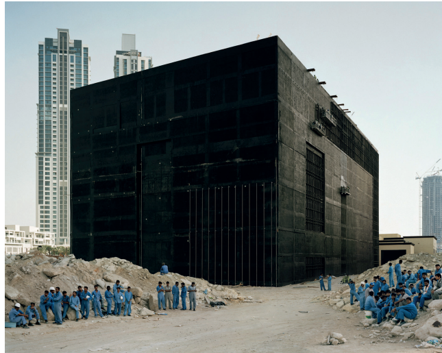
Watercooling Plant, Bas Princen, Dubai, 2009
