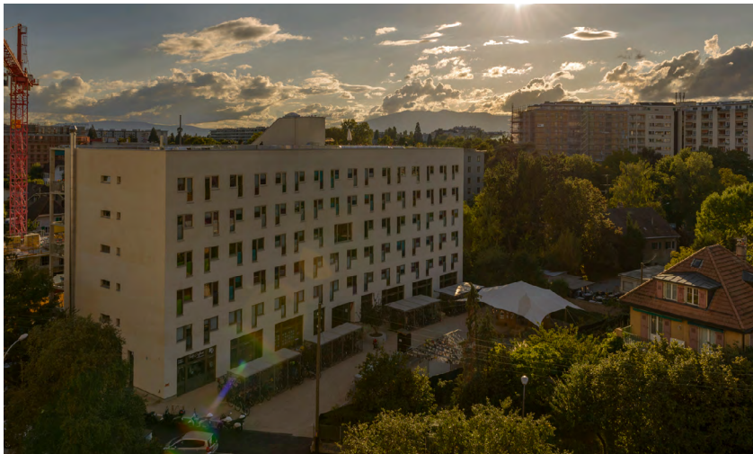
Fig.9 Photo Façade Sud, Soubeyran © atba
