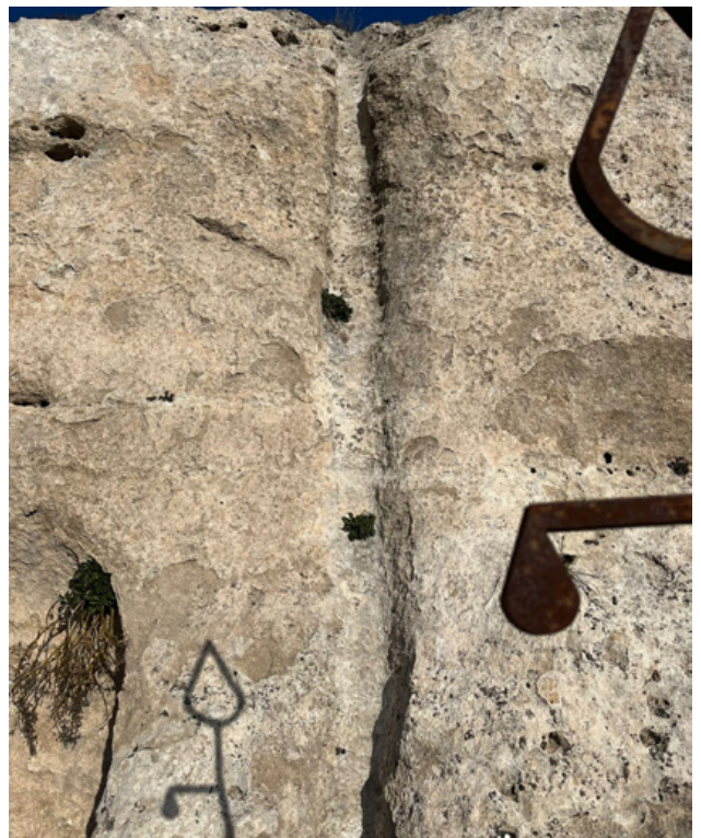
Fig. 86 Channel in the cliff to transport and collect rainwater
