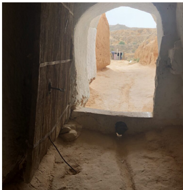
Fig. 55 Trench to collect reain water
