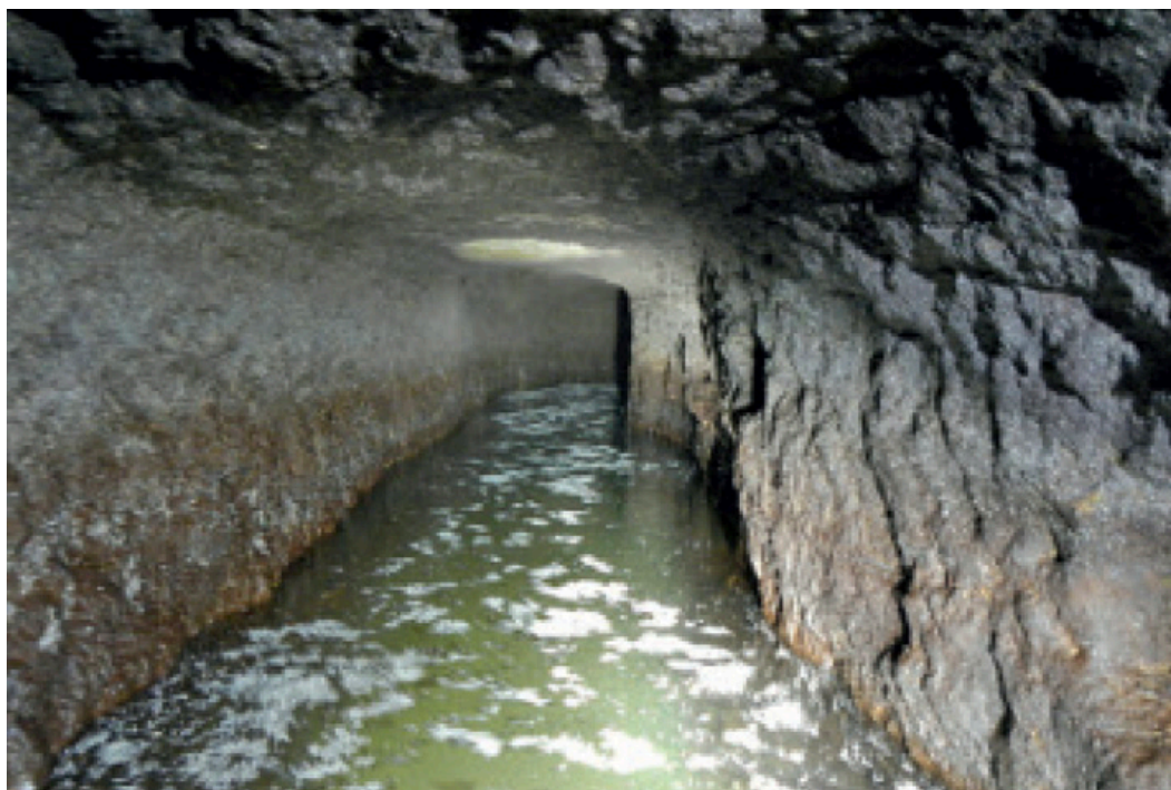
Fig. 123 Belvedere tunnel- cistern, still flooded in a period of drought.
