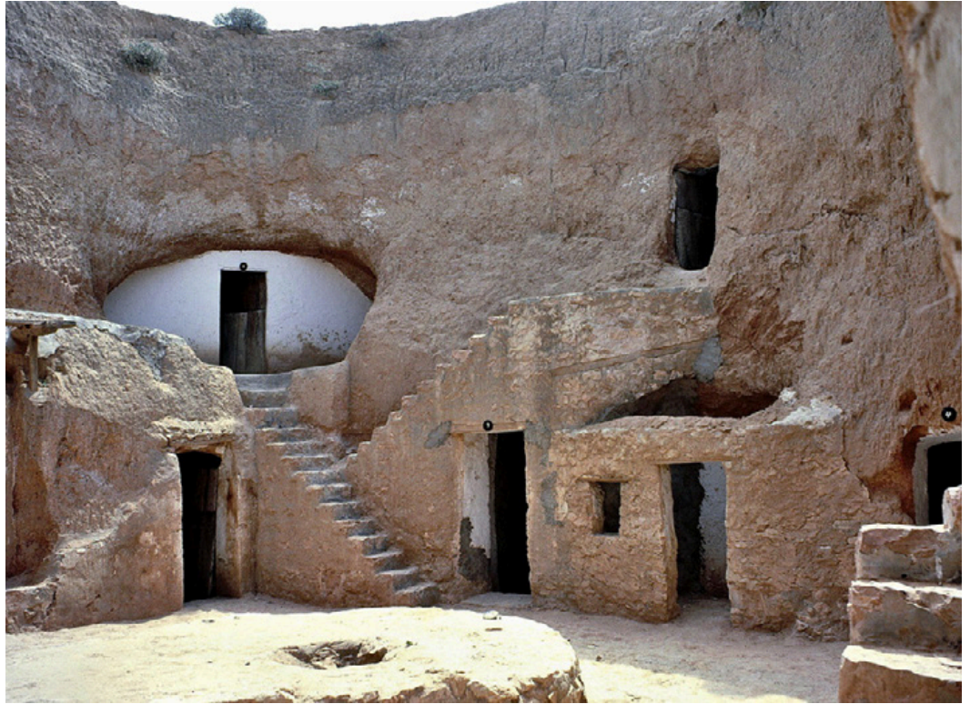
Fig. 38 Stairs to access on the upperfloor
