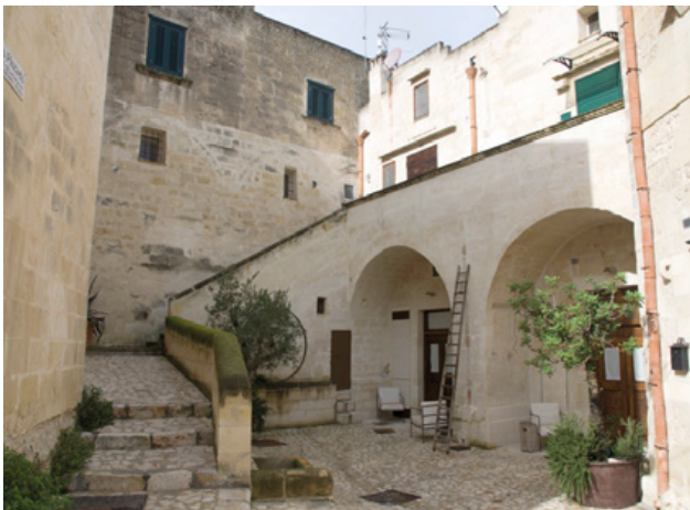
Fig. 67 House with access from the courtyard
