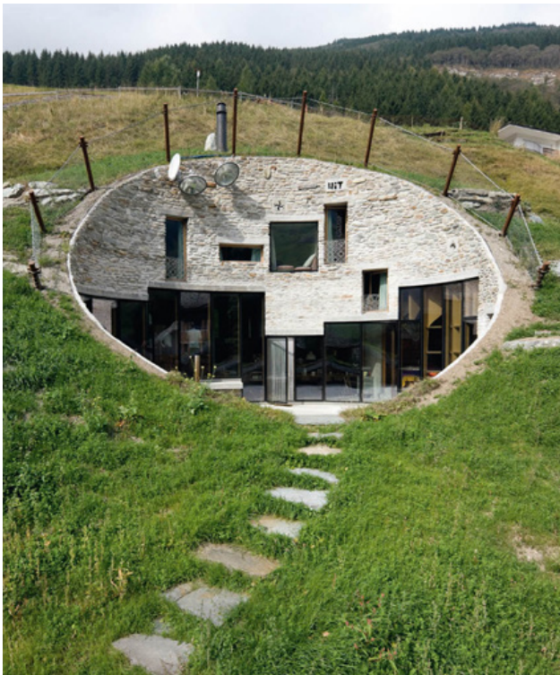
Fig. 21 Picture of the facade of Villa Vals
