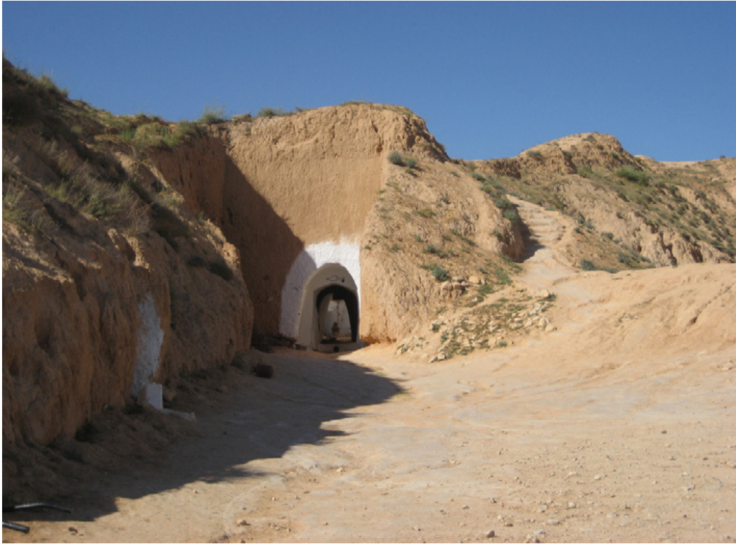
Fig. 36 View of an access corridor
