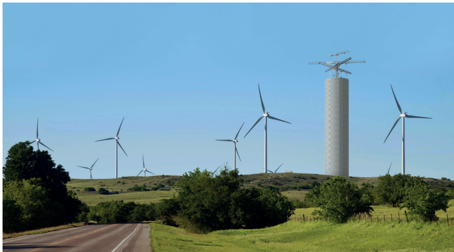
13. Energy Vault storage tower + co-located with wind farm. Developed by Swiss start-up. First prototype built in Castione, Ticino, Switzerland. (ongoing)
