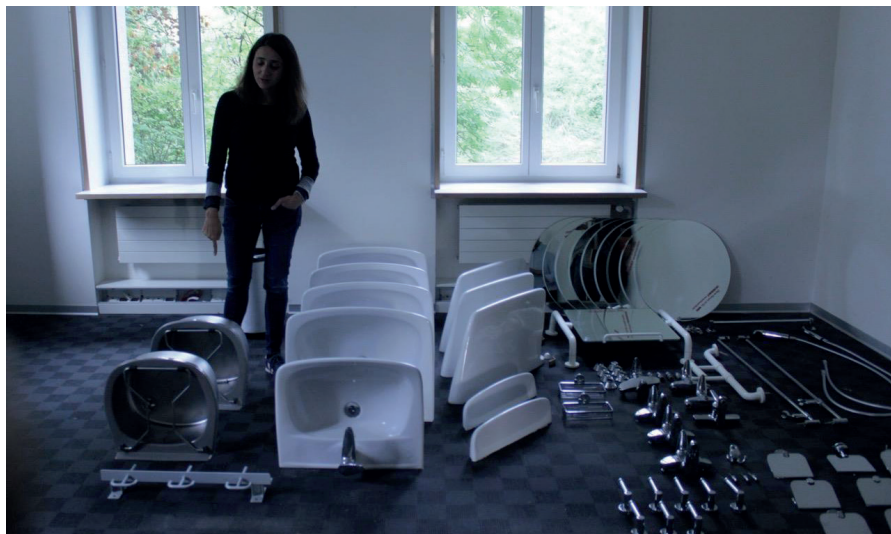
9. Dismantling of building materials in the headquarters of SIG Areal, in Schaffhausen for it reuse. Workshop Deconstruction - CAS, ETH Zurich
