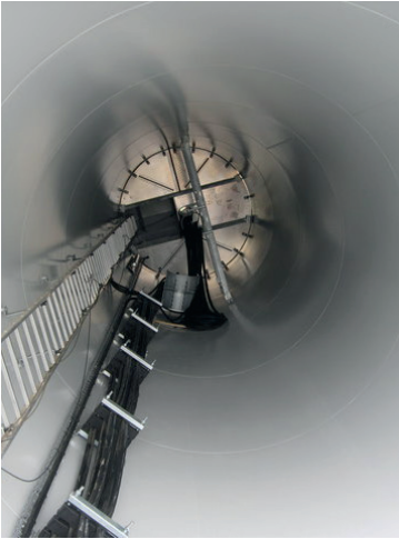
5. Inside Turbine Tower
