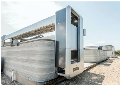
4. Concrete printing houses from ICON
