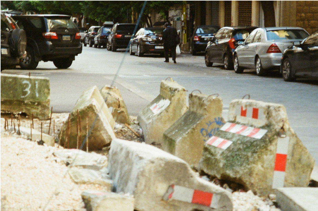
Figure 17 The idewalk project's unfinished construction site
