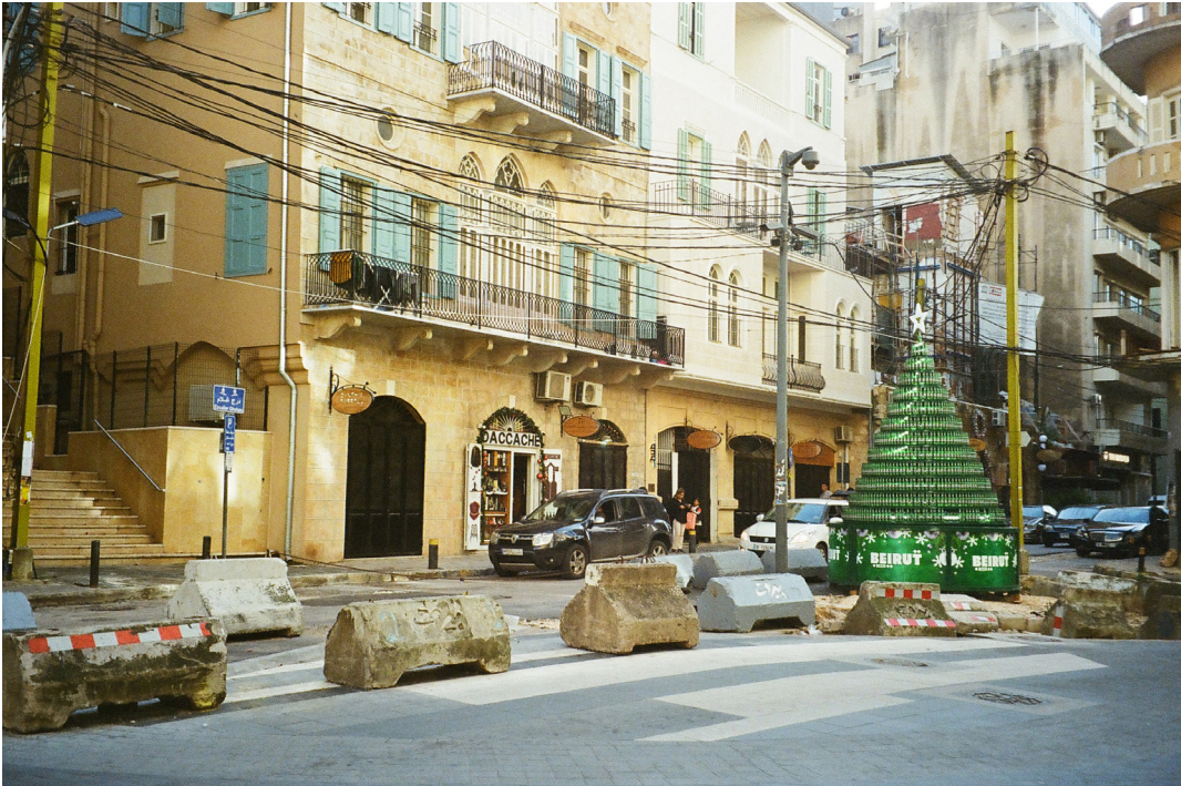
Figure 16 Sidewalk project unfinished site, with the staircase leading to the Mukhtar’s office on the left. The staircase is named after the Mukhtar ‘Gholam.’
