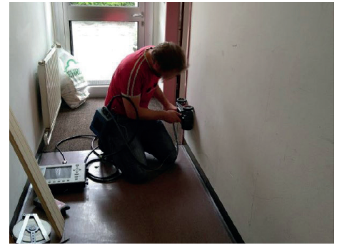
Scan GPR d'un mur intérieur ©Kovacic & Honic Scanning and data capturing for BIM-supported Ressources assessment: a case study
