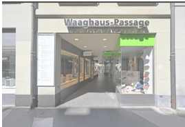
Waaghaus-Passage 8 apartment 3rd floor 88 m2
