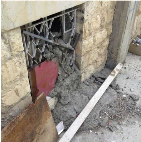
Figure 68 : « Mu'taz Ibrahim Khalil Hijazi's window before the hose was introduced to pour the cement »
