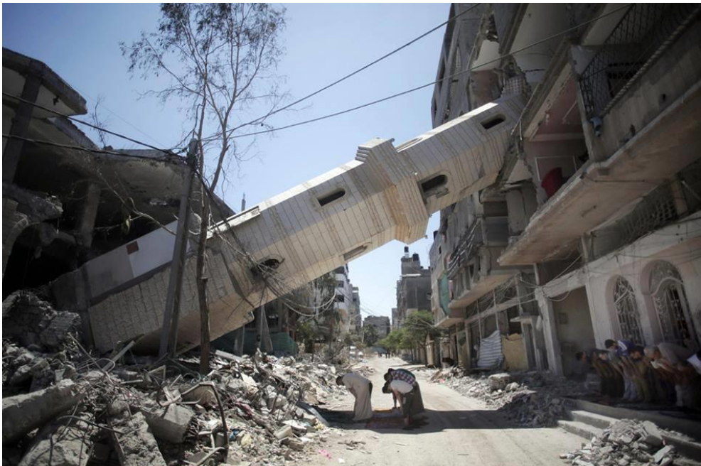
Figure 14: Minaret of Soussi mosque toppled by Israeli strikes in Gaza city, 2014 ©AP/Khalil Hamra
