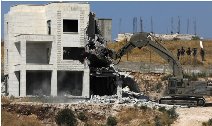
Figure 27: Demolition with shear attachment
