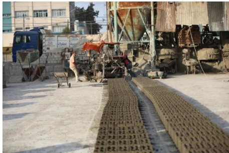
Figure 18: "Concrete blocks are made from the remains of destroyed homes after recycling" ©Ashraf Amra/ Al Jazeera
