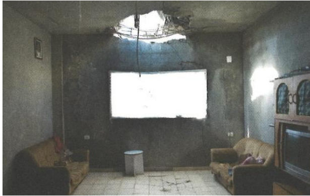
Figure 33: House struck by drone in North Gaza, Kent Klich
