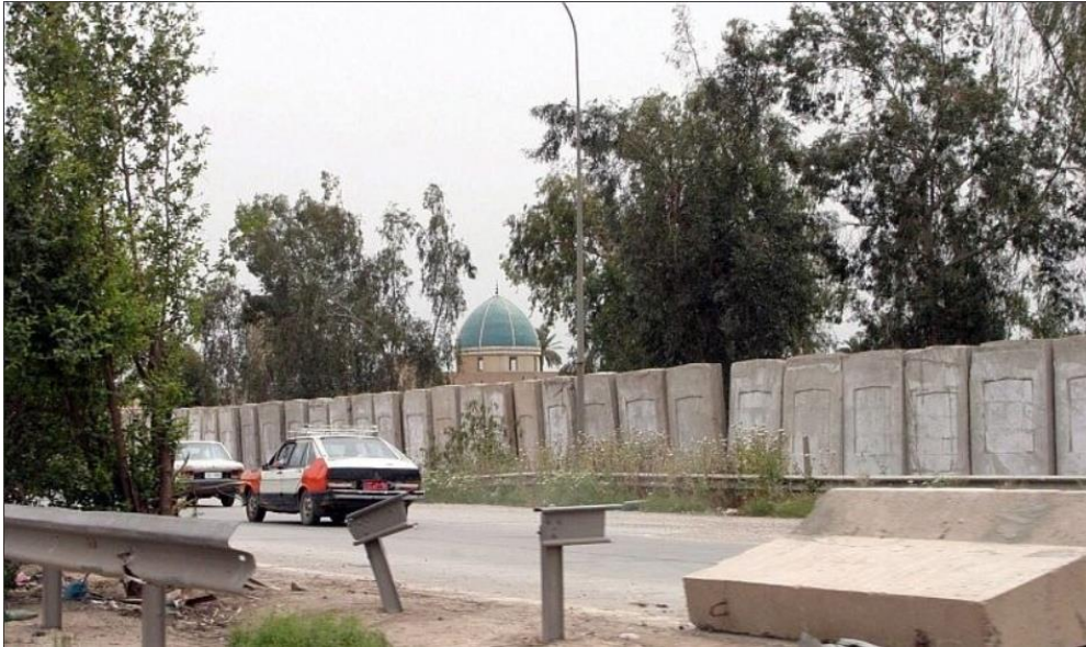
Figure 52: Part of a concrete wall in Al Adhamiya, a district in Baghdad
