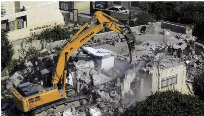
Figure 28: Demolition with hydraulic hammer
