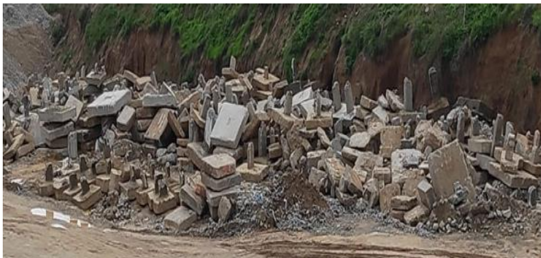
Figure 20: Large concrete blocks and foundation elements sorted out from rubble
