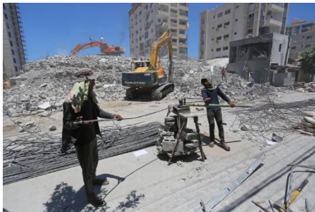
Figure 19: "Palestinian workers modify steel rods for the construction of buildings destroyed by Israeli fighter jets during the recent attacks on the Gaza Strip "©Ashraf Amra/ Al Jazeera
