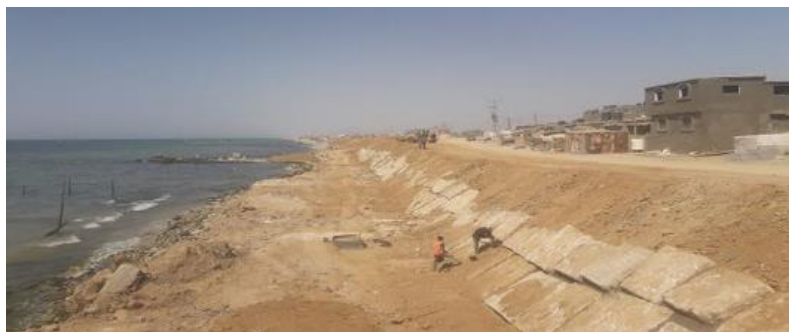
Figure 21_ Foundation blocks reused for shoreline protection in Gaza Beach
