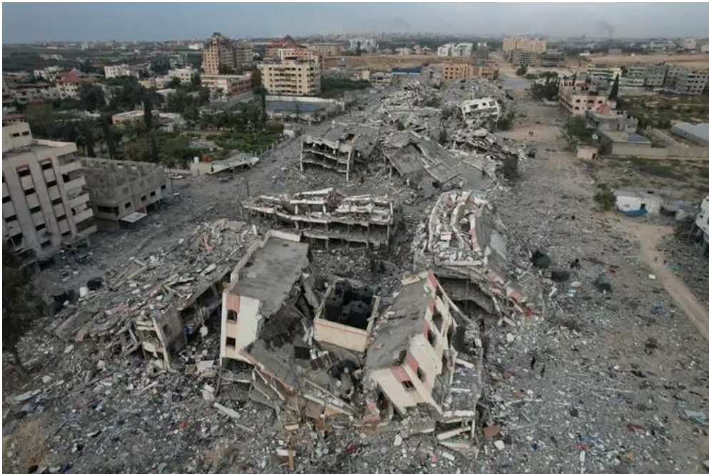
Figure 7: "An aerial view of heavily damaged, collapsed buildings caused by Israeli attacks during the 4-day humanitarian pause at Al-Zabra region in Gaza City, Gaza on November 25, 2023."
