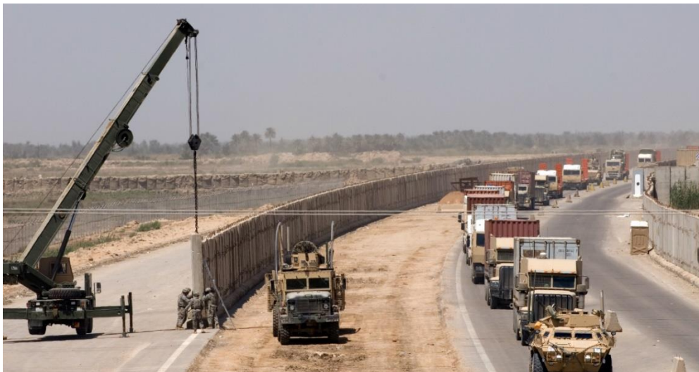
Figure 53: Deployment of concrete wall in Iraq Image credit: Spc. Kiyoshi Freeman, US Army
