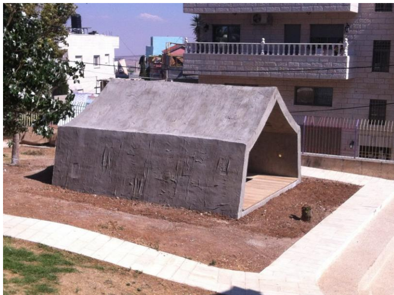
Figure 48: Concrete tent exterior
