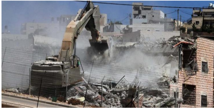
Figure 26: House demolition with shovel attachment
