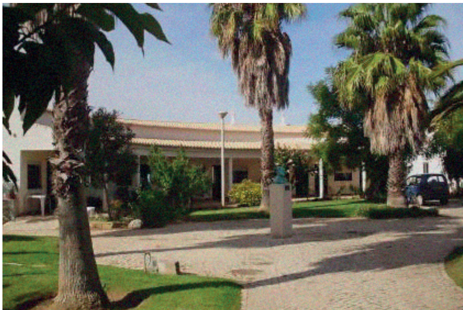
Above: Monte Da Palhagueira, Algarve. Nursing home, church, swimming pools and greens of golf like a permanent holidays resort. Below: São José de Alcalar, Algarve. Built in 1989, this home-village gets closer to the co-housing concept for senior with its 52 appartments.
