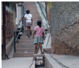
fig. 85 - urban stairs coupled with a rain water drain
