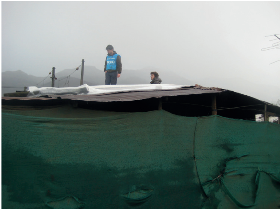
fig. 88 - architecture students (with whom I worked) repairing roofs with the NGO TECHO in campamentos during floods in Santiago, Chile
