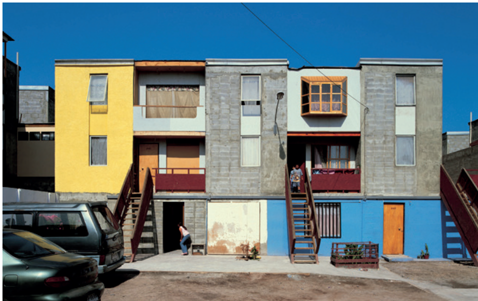
fig. 67 - after the expansion of the families within the structural frame. Unfortunately due to the high price of land and the size of the parcel, a big part of the public spaces is for parking
