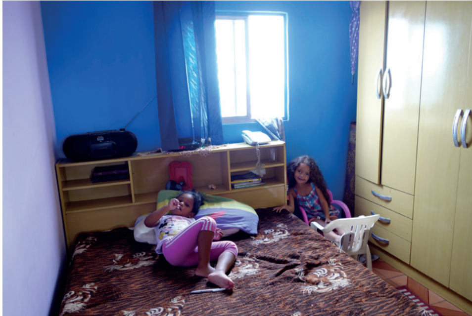
fig. 46 - the quality of the rooms vary widely from luminous to dark with water infiltrations
