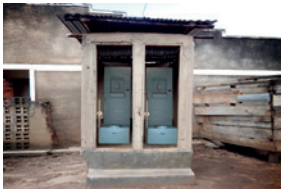
fig. 80 - dry toilets retrofitted in latrin pit
