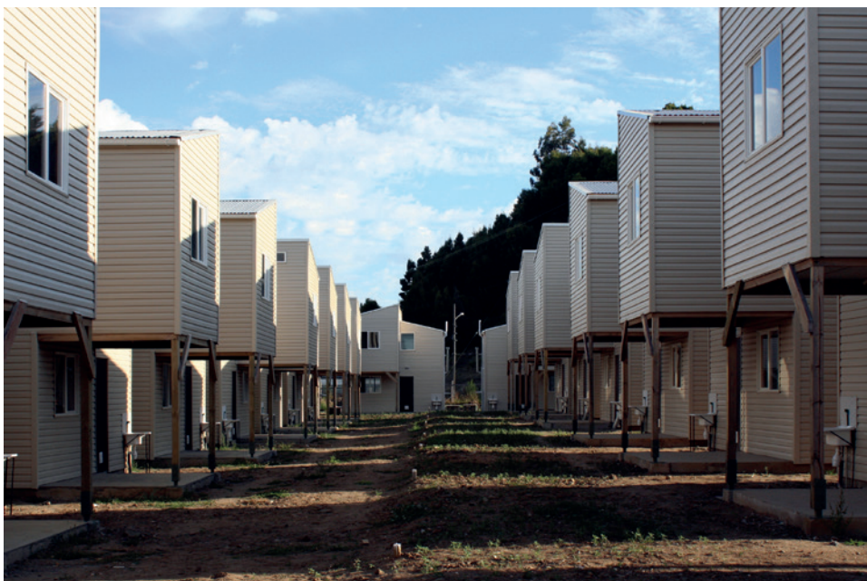
fig. 61 - a basic structure and a concrete slab are ready for the inhabitants to build expansions. The repetition reduces construction costs.
