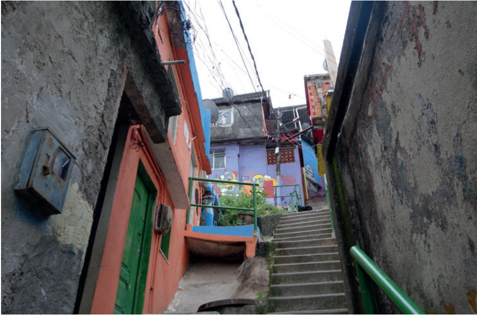
fig. 35 - a typical stairway that connects the house entrances
