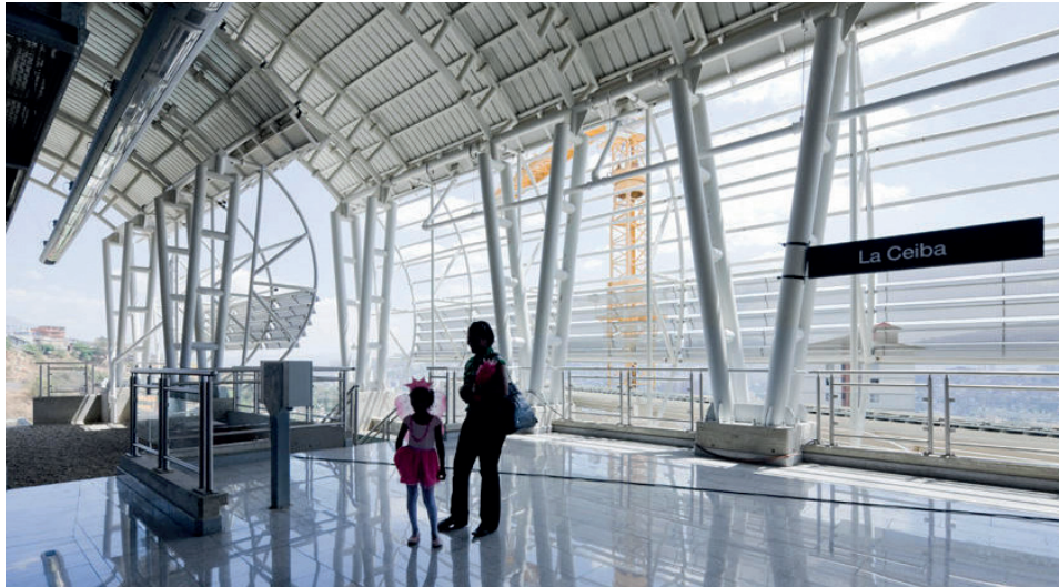
fig. 71 - the end stations connect to the existing metro line and become extensions of it. The visibility and feeling of security the metro cable brings has had the effective impact of dropping criminality down by 30%. 121
