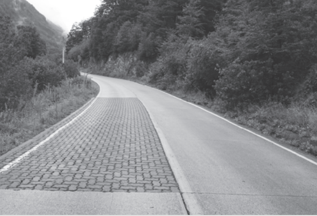
Hybridation asphalte-pavés Puerto Aysén
