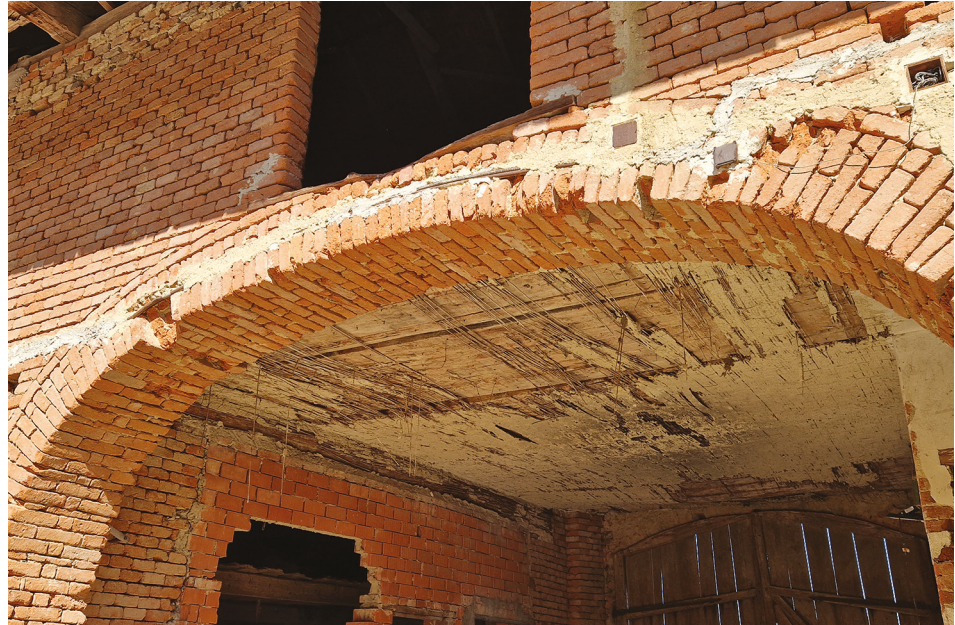
Figure 05.05 Old, handmade bricks and adobe-wooden floor construction; Frau Huber's Vierkanterhof (Ürmössy, 2023)
