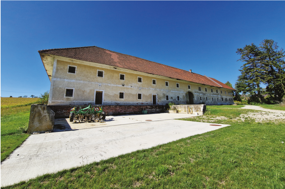
Figure 08.02 South-eastern external facade of "Leebgut" Vierkanterhof; water and sewage system organised below concrete deck in the front (Ürmössy, 2023)
