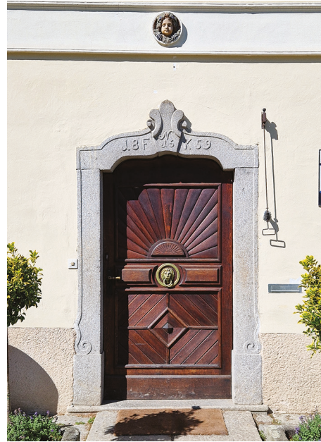
Figure 04.19 Doors of the facade of Sumerauerhof Vierkanterhof Museum: [Left] main granite door for carriages; [Right] entrance of the Mittelflur (Ürmössy, 2023)
