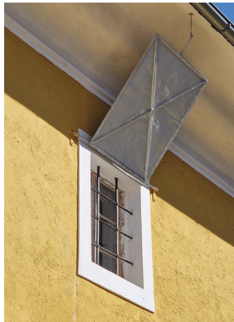
Figure 04.21 Facade of Sumerauerhof Vierkanterhof Museum: (Left) window on courtyard facade with fire-proofing latch covering; (Right) Sgraffito decoration technique on Backhaus next to the Vierkanterhof (Ürmössy, 2023)
