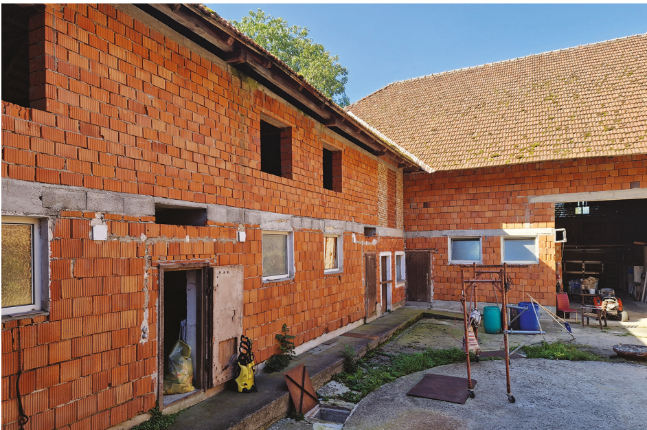
Figure 05.04 Bricks from the 1980s and 1990s with concrete floorplans and lintels; Frau Huber's Vierkanterhof (Ürmössy, 2023)
