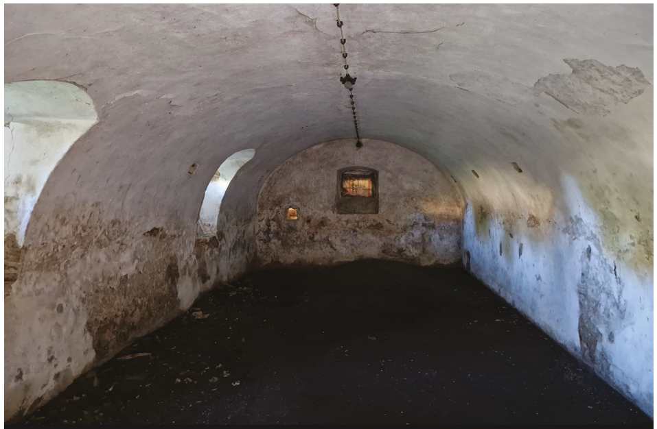
Figure 08.11 Apple and pear cider storage cellar in small building next to "Leebgut" Vierkanterhof; room in cellar with shaft lights (Ürmössy, 2023)
