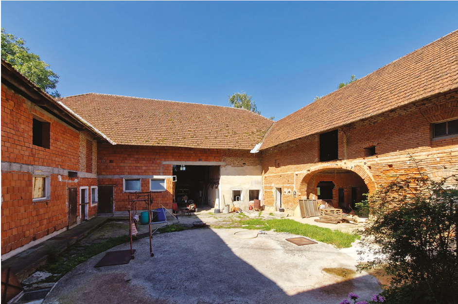
Figure 05.03 Courtyard under renovation, exposed brick telling the history of the structure; Frau Huber's Vierkanterhof (Ürmössy, 2023)
