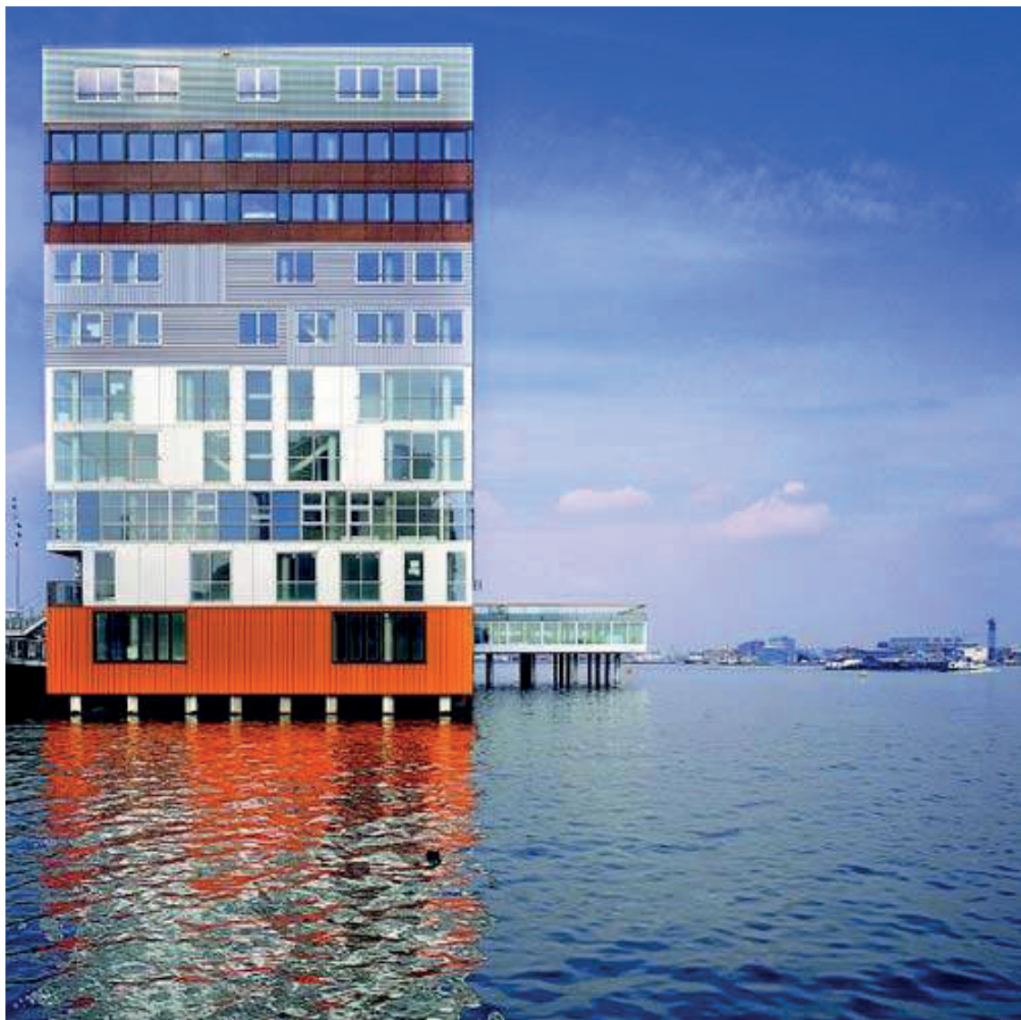
MVRDV, Silodam Building , Amsterdam, 2003
