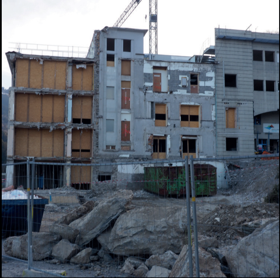
deconstruction of the east wing of Monthey hospital, providing re-used insulation and concrete
