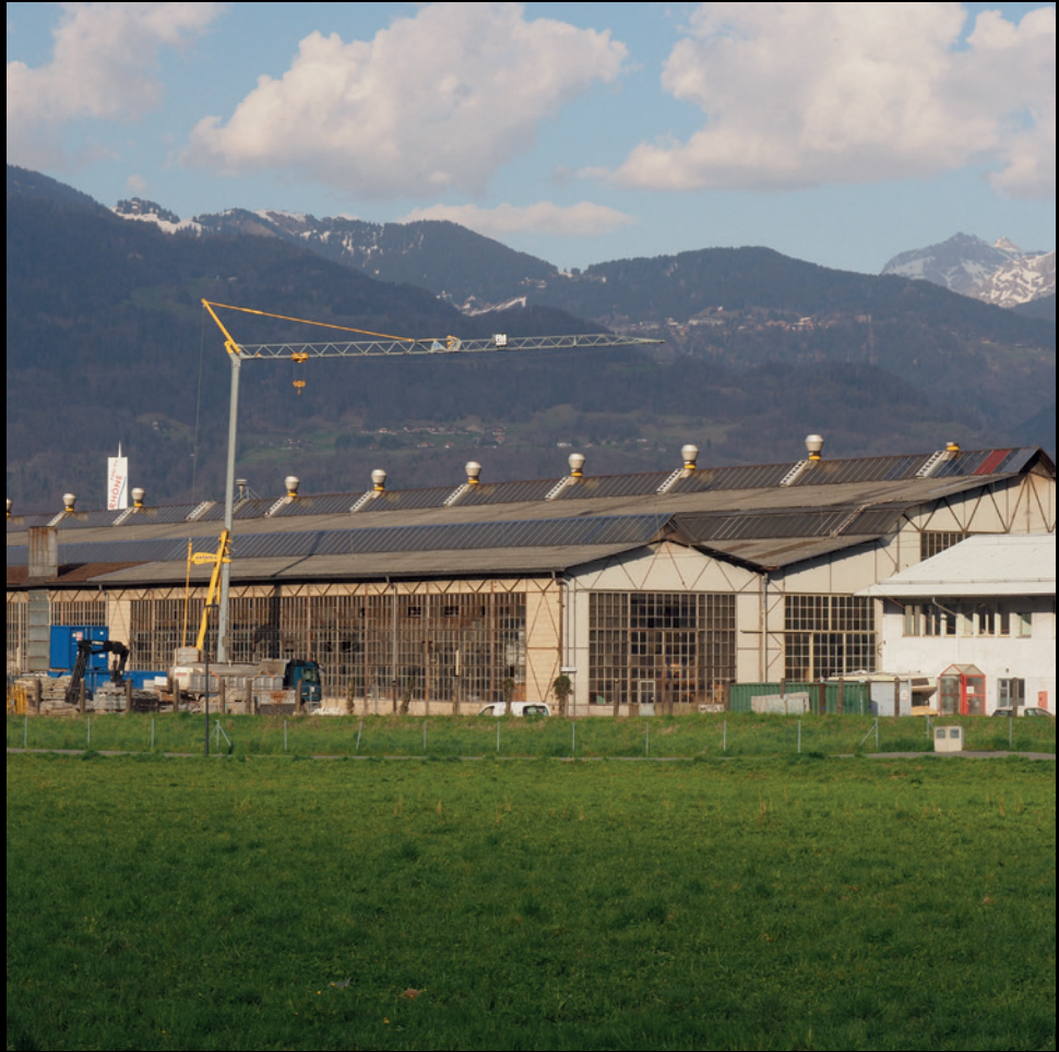
deconstruction of industrial sheds in Monthey, providing corrugated metallic and transparent PVC plates
