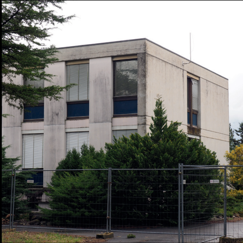
administrative buildings + technical buildings : prefab + cast concrete
