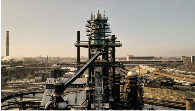
Figure 6.8. Blast furnace no. 1 (bolt tower) drone image
