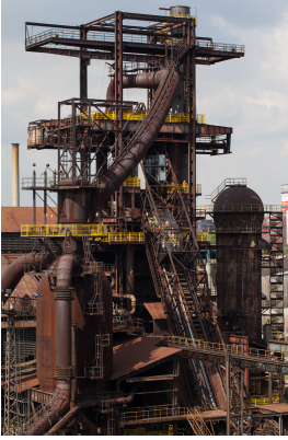
Figure 6.9. lifting platform of the BFi transformed into a visit eleva- tor(@Josef Pleskot, apatelier)
