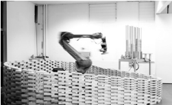
Computer-assisted robotic bricklaying
