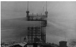
Stockholm Telephone Tower
