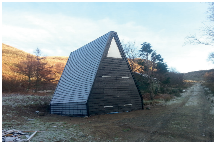
Wikihouse A-barn completed project
