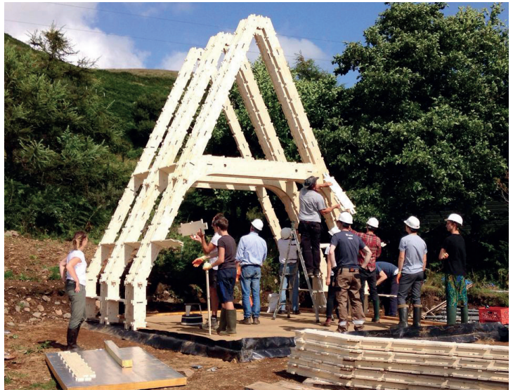
Wikihouse fast profiles construction
