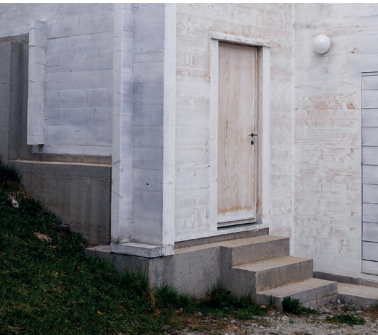
[Fig. 45] Lower entrance with its distinct threshold, concrete pedestal, and 'strickbau' corner detailing
