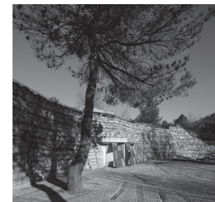
[Fig. 49] The dry stone wall and timber railway sleepers set into the concrete ground surface
