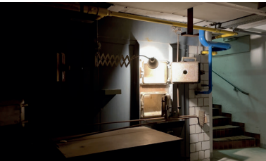
[Fig. 36] Crematorium technical basement: an old oven
