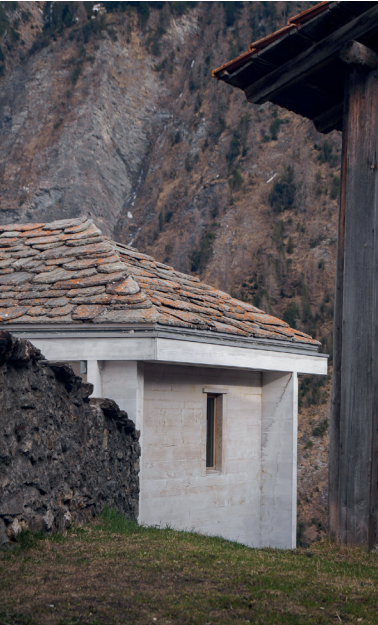
[Fig. 42] Back access to the lower entrance
