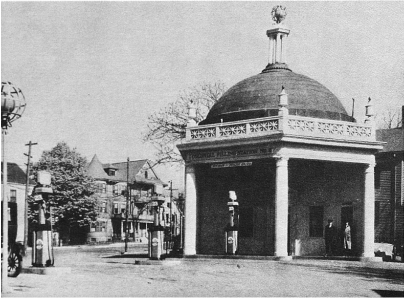
Fig 1.20 Station type de la chaine Beacon Oil, Dorchester, Massachusetts.
