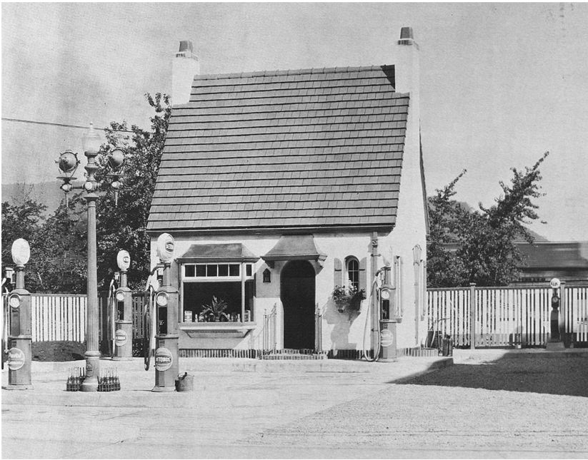
Fig 1.13 Petite station essence style 'English cottage' à Binghamton, New York.
