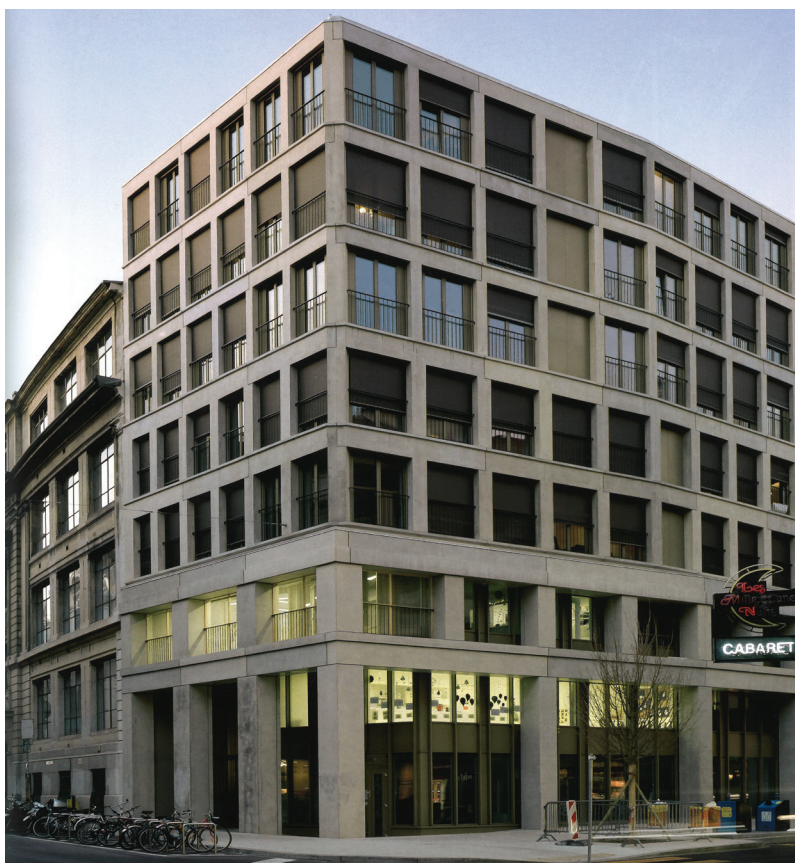
Fig|15| Sergison Bates architect, Novartis Welcome Center and Office, Façade.
