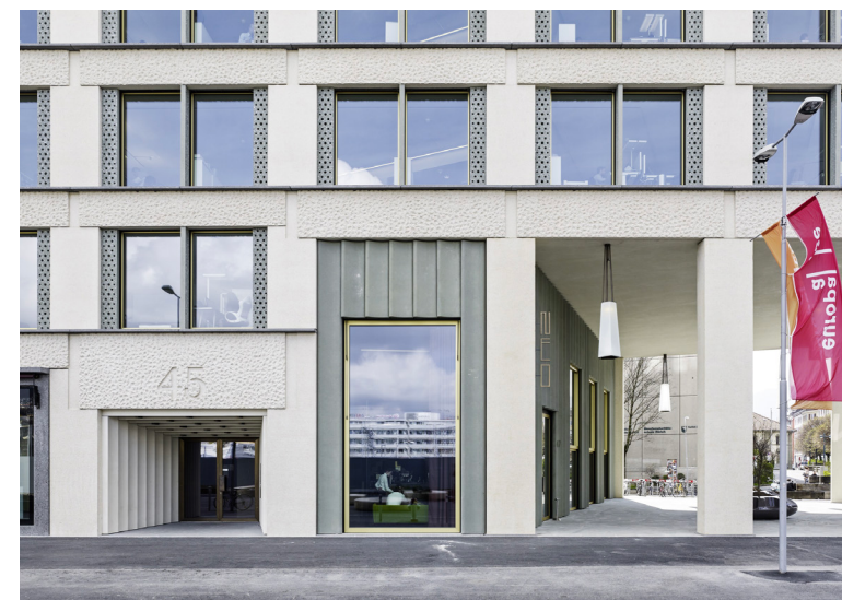
Europaallee Mixed-use Building, Zurich, ©Caruso St John
