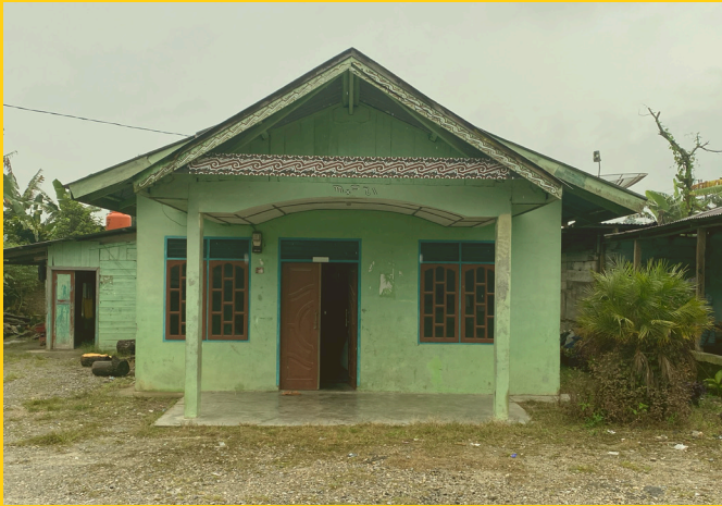
Main entrance of rumah Uda .
