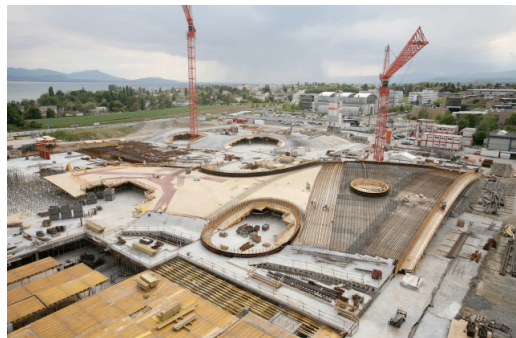
Construction du Rolex Learning Center
