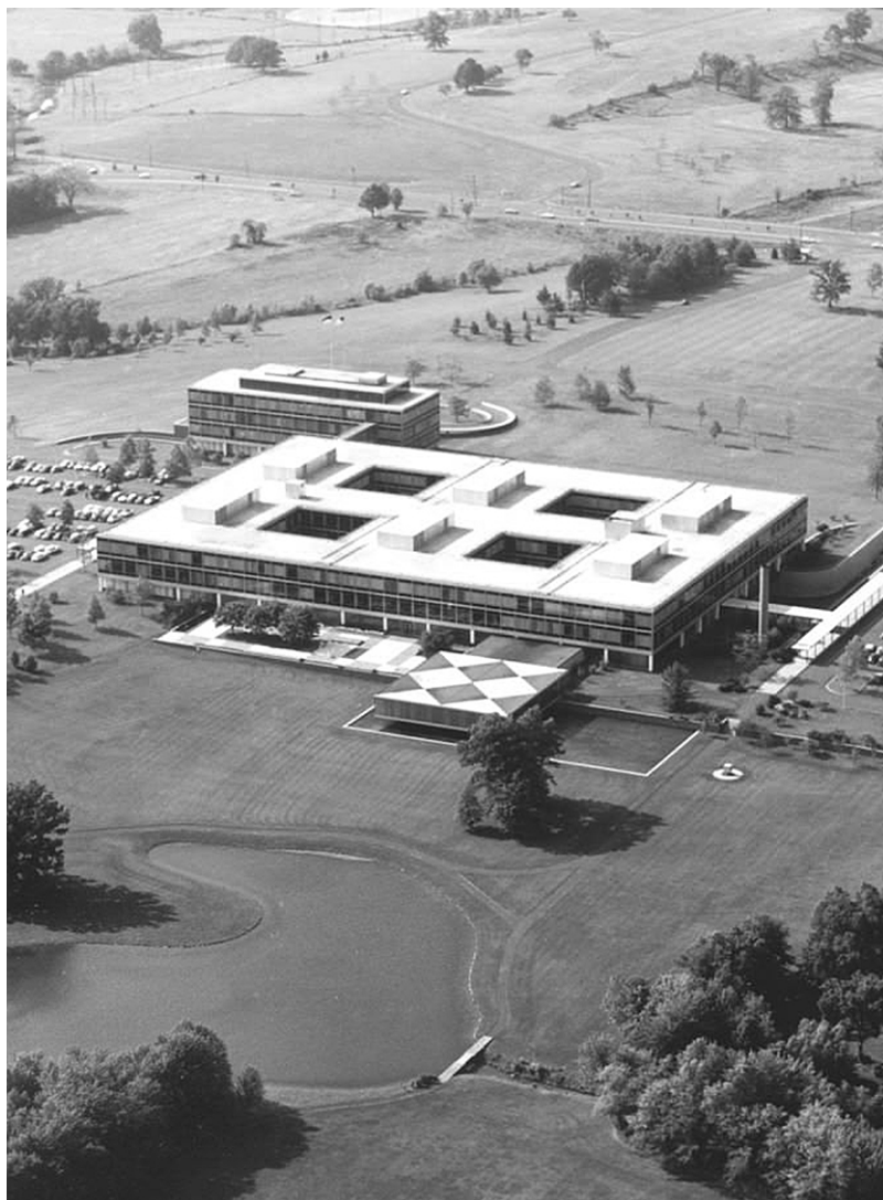
Fig 20. Skidmore, Owings and Merrill (SOM), Connecticut General Life Insurance Company, Bloomfield, Connecticut (USA), 1954-57
