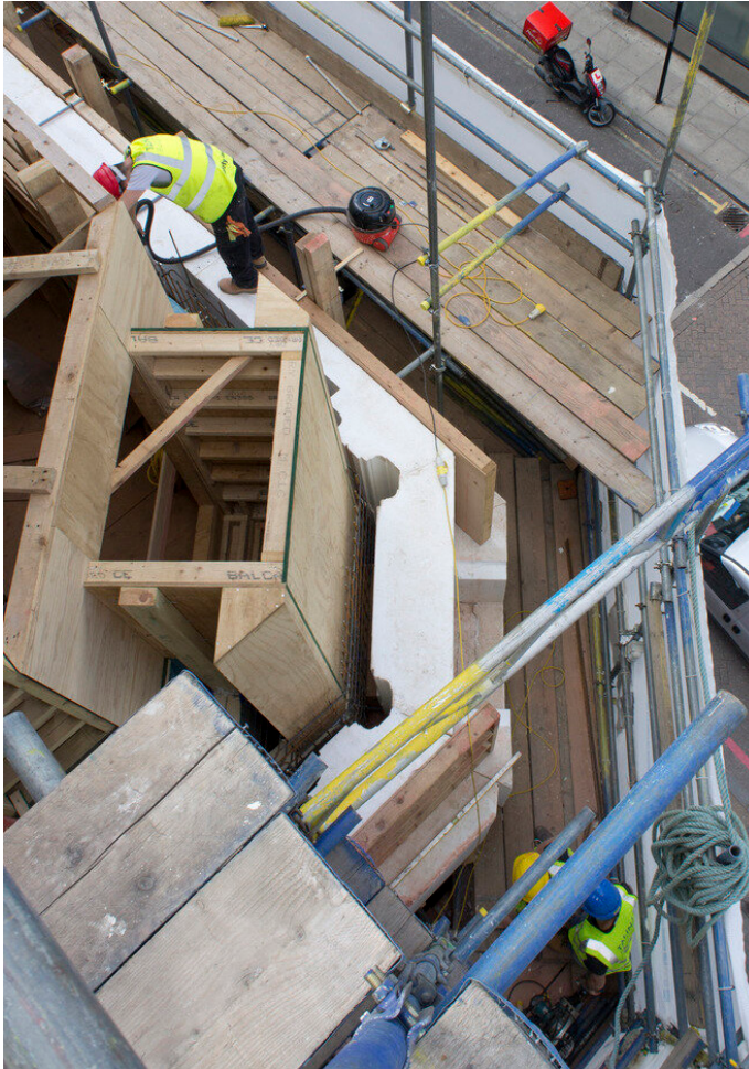
Figure 18. Construction on site, photograph by Timothy Soar, 2017.
