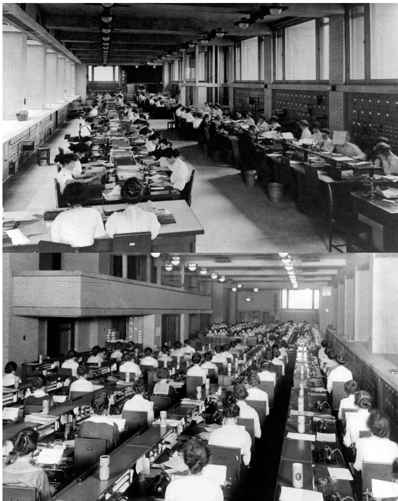
Fig 7. Frank Lloyd Wright, Larkin Building, Buffalo, New York (USA), 1904-06.
