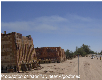
Production of "ladrillo", near Algodones
