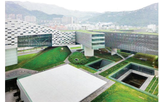
figure 35 : Horizontal Skyscraper de Steven Holl Architects à Shenzhen , Holl, Steven, & A+T Ediciones. (2014). This is hybrid : An analysis of mixed-use buildings . Vitoria-Gasteiz, Spain : A+t architecture, pages 123
