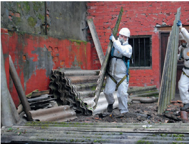
Figure 22. Photography of workers removing components contaminated by asbestos
