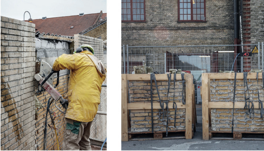
Figure 27. Photographies by Lendager Group, worker cutting up brick modules and modules ready to be transported
