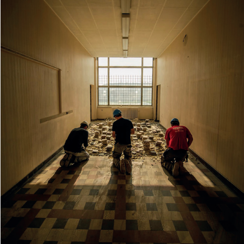
Figure 9. Photography by Olivier Beart, careful dismantlement to recover the tiles
