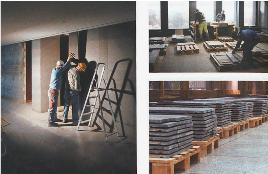
Figure 12. Photographies by Rotor, a few steps of a deconstruction process: dismantling, cleaning and sorting on pallets
