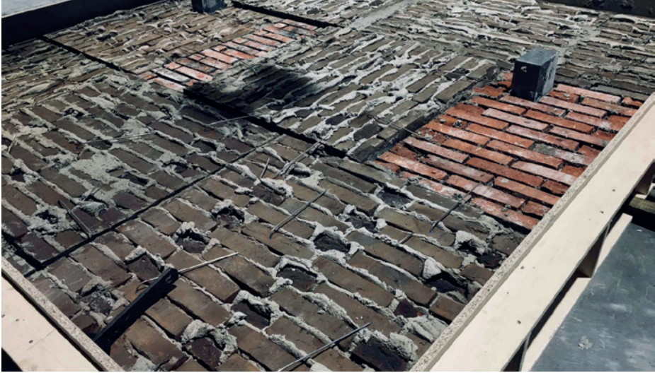
Figure 28. Photography by Lendager Group, production of the brick module
