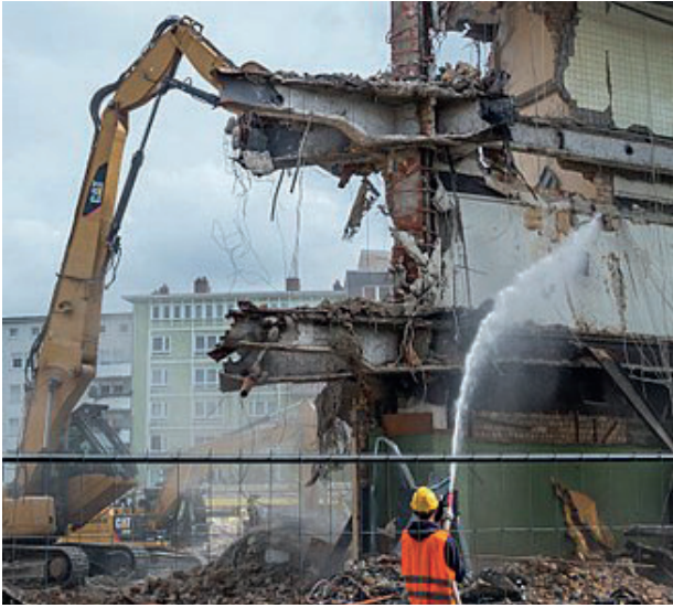
Figure 5. Photography of a building's demolition
