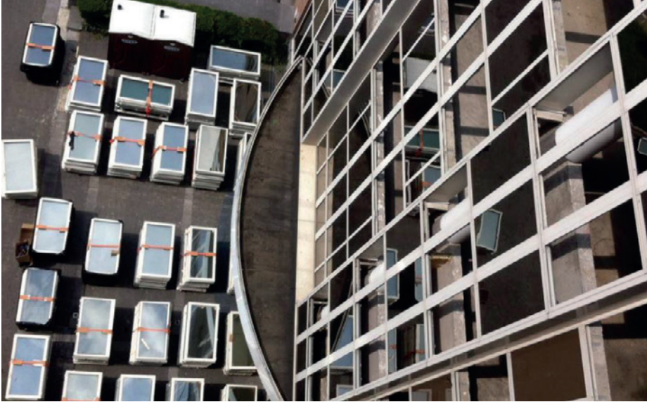
Figure 13. Photography by Stephan Kampelmann, disassembly and preparation of window frame on pallets, 2017
