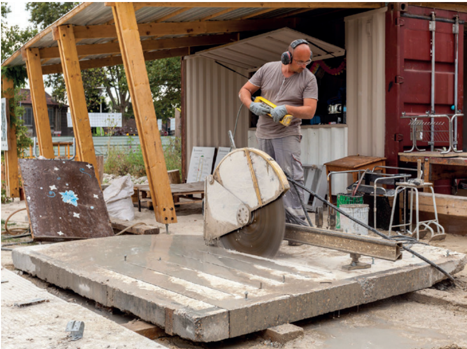
Figure 42. Photography by Alexis Leclercq, pieces of slabs recovered from the demolition are sawn on site
