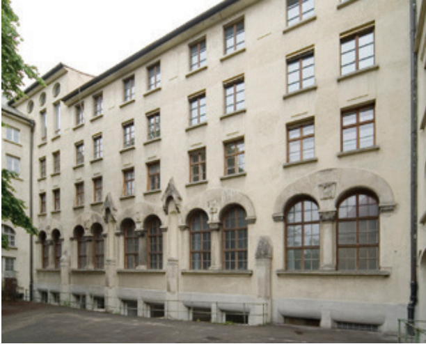
Figure 39. Photography by Hild und K Architekten, original building before demolition
