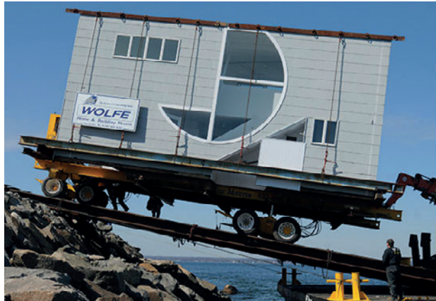
Figure 7. Photography by Rob Bennett, transportation of the Nathaniel Lieb house onto a barge
