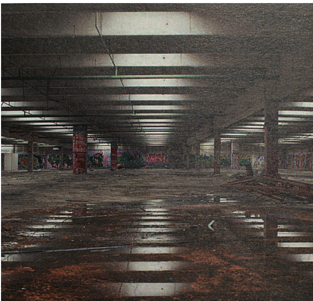
Figure 16. Photography by Thomas Béhuret, “93450 Mutations”, the Printemps warehouse before demolition
