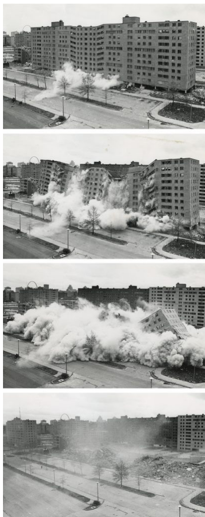
Figure 53. Pruitt-Igoe, Demolition of one of the buildings.
