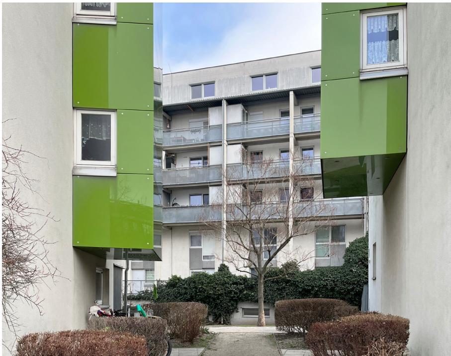
Site view of Frauen-Werk-Stadt – unit B in the foreground and unit A in the background. Photo by the author, 2023.
