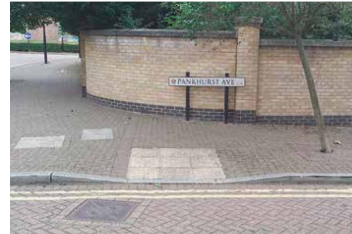
A "dropped curb" or "pram ramp". Standardised urban feature created by Selwyn Goldwin, author of Universal Design: A Manual of Practical Guidance for Architects , 2000
