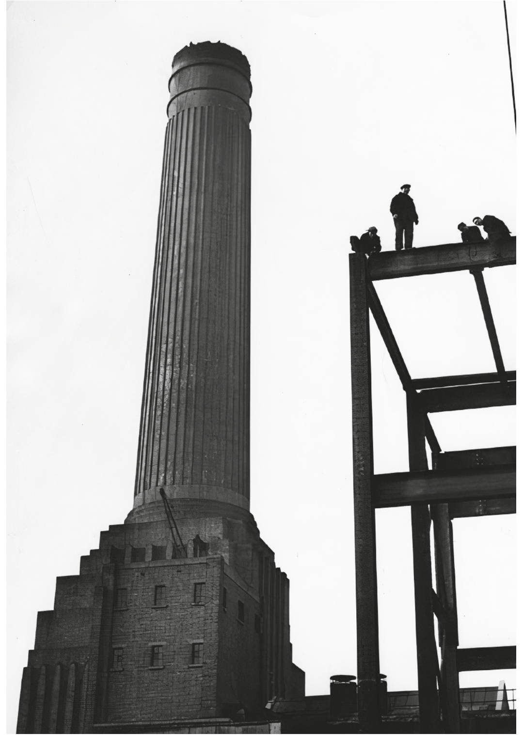
Fig. 17: Chimney's scaffolding, 1951. © Fox Photos / Getty Images.
