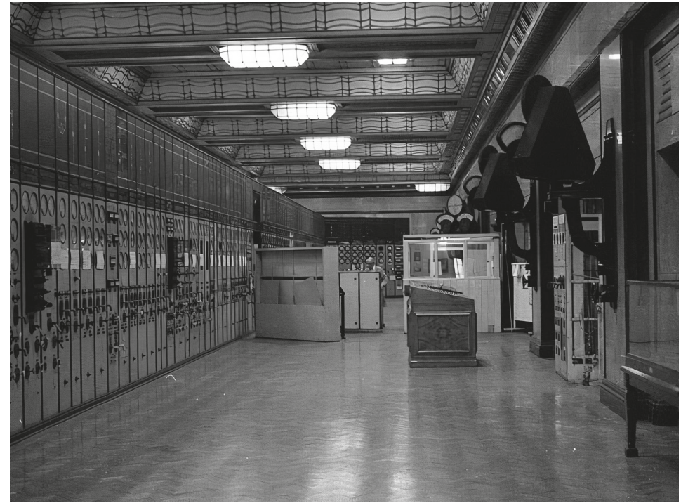
Fig. 7: Switch House A, © Ian Lidell.
