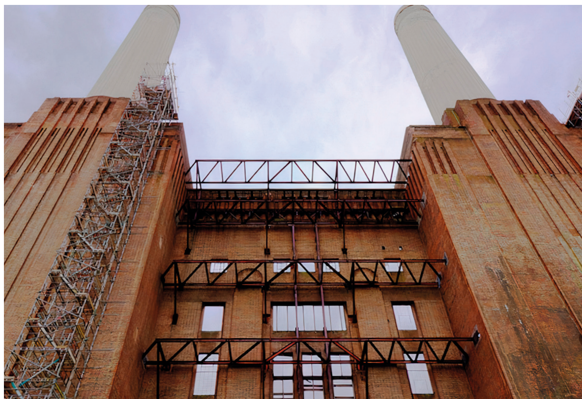
Fig. 31: Opened structure of Battersea Power Station, 2016, MessyNessyChic.
