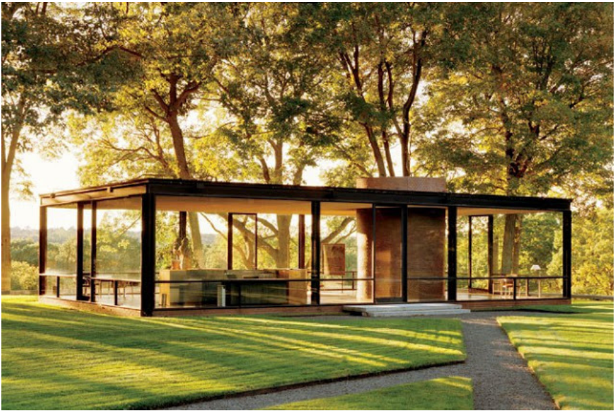
[9] Glass House , Philip Johnson, New Canaan, USA, 1949 (Inconnu, 2013)
