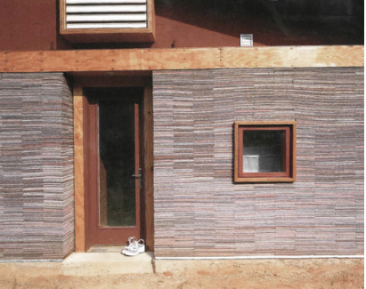
Façade sud, Lucy Carpet House © Rural Studio
