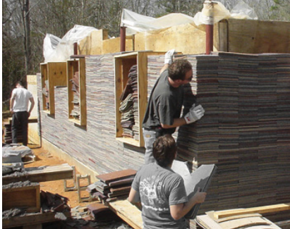
Construction de la Lucy Carpet House © Rural Studio
