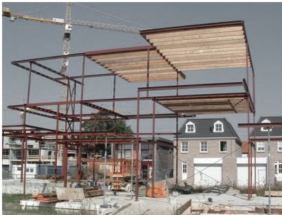
Structure porteuse, Villa Welpeloo © Superuse Studios
